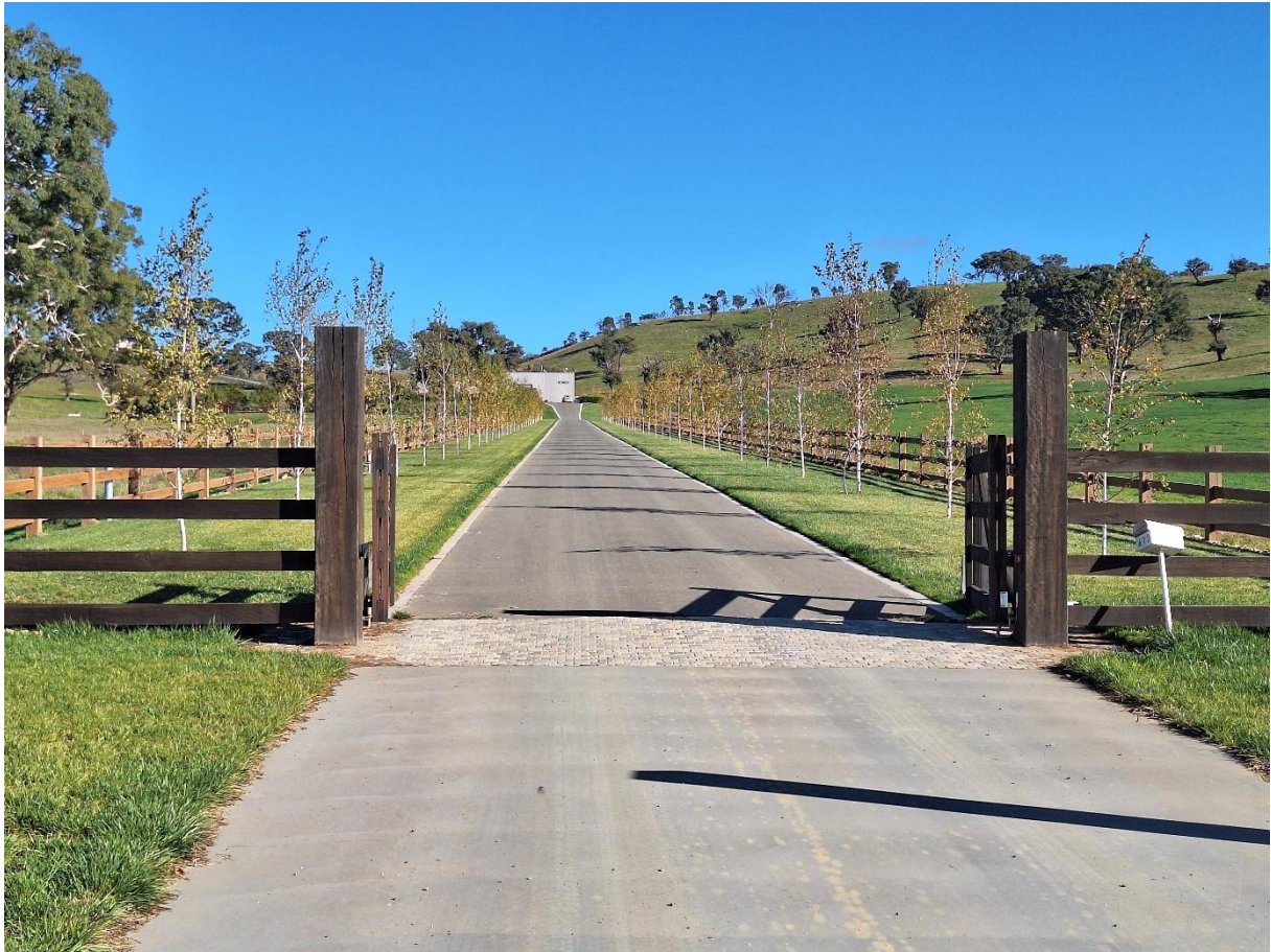
Plate 8: The existing access to PL-2
